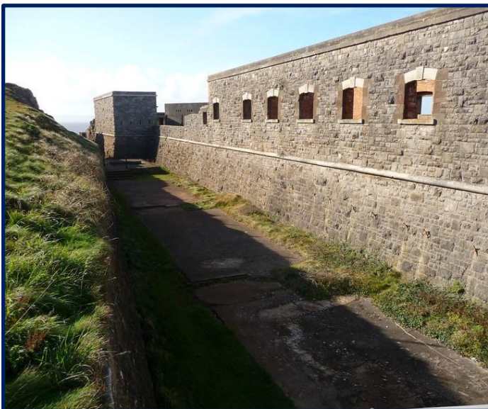
A trench outside the Victorian fort © Chris Talbot
