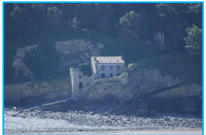
A derelict building on Steep Holm © Ben Hollier
