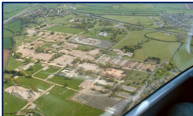
The site of RAF Locking after demolition © Steve Pemberton
