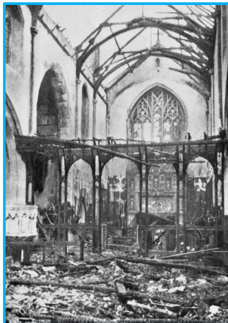
Bomb damage at St. Paul's Church © Weston-super-Mare Library
