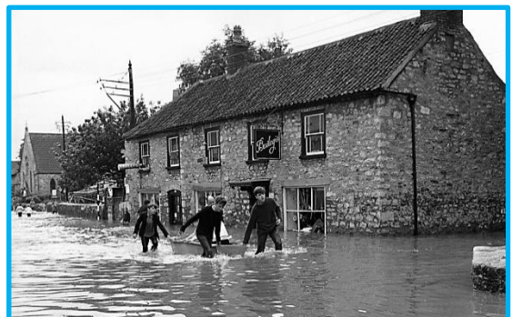
Flooding in Congresbury, 1968 © Weston Mercury
