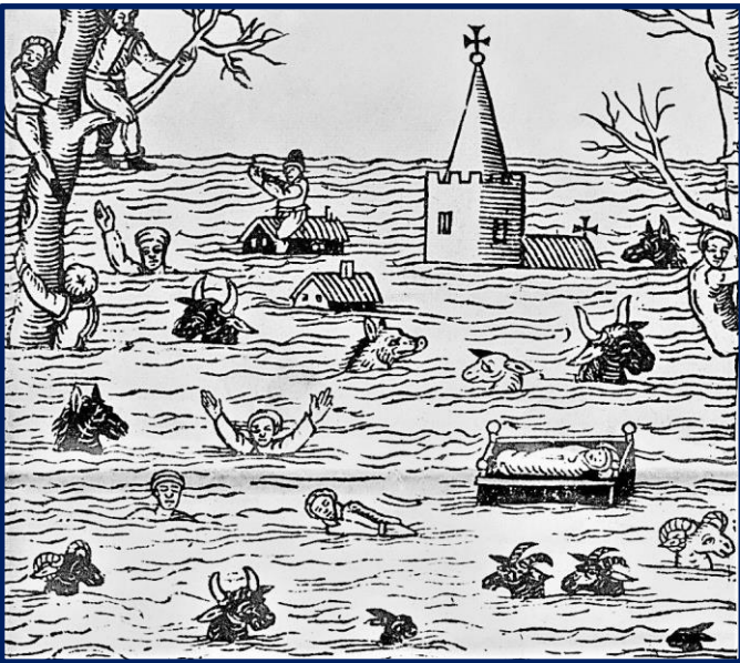
A drawing showing the devastation caused by the flood of 1607
