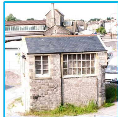
The original Bristol & Exeter Railway signal box © Geof Sheppard
