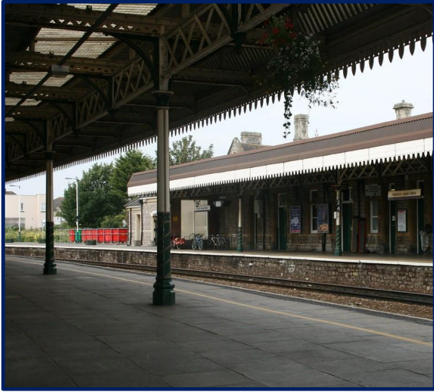
Weston's current station, built in 1884 ©James F Clay
